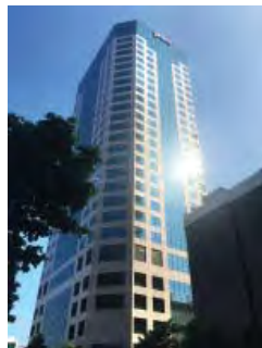
◀ PWC Building Cross Street S$746.8M/US$534.31M in February
