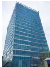
◀ International Metropolis Plaza Building 3 Pudong RMB2.5B/US$379.0M in August
