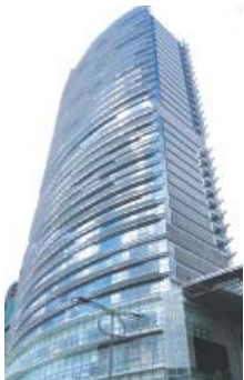
▼ The Ascent Petaling Jaya, Selangor RM347M/US$82.2M in July
