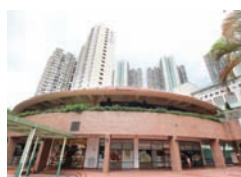
◀ Ka Fuk Shopping Centre & Carparks Fanling HK$588.3M/US$75.9M in October
