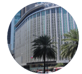
INSULAR LIFE MAKATI BUILDING ↗
